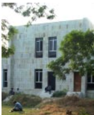
New Library Building
